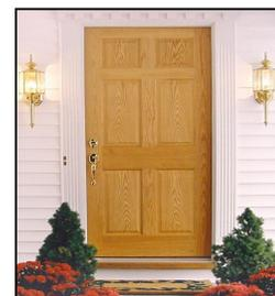
Consists of stiles, rails and one or more panels, the stiles and rails forming the frame around the panel; "stile and rail" door.
